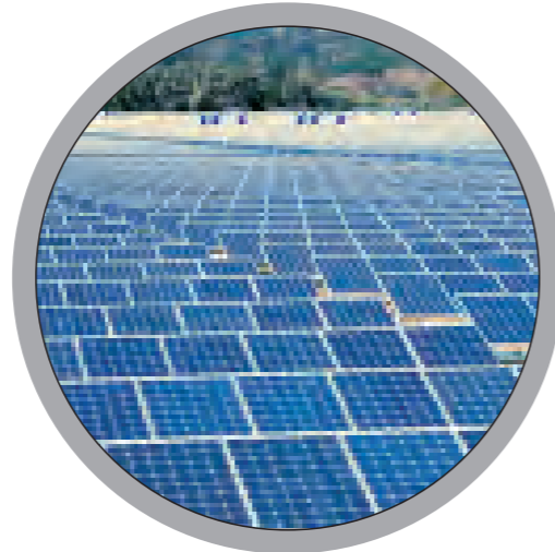
Solar Power System
